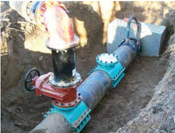
Typical 18" x 12" folding head line stop operation with separate bypass on sewage force main
